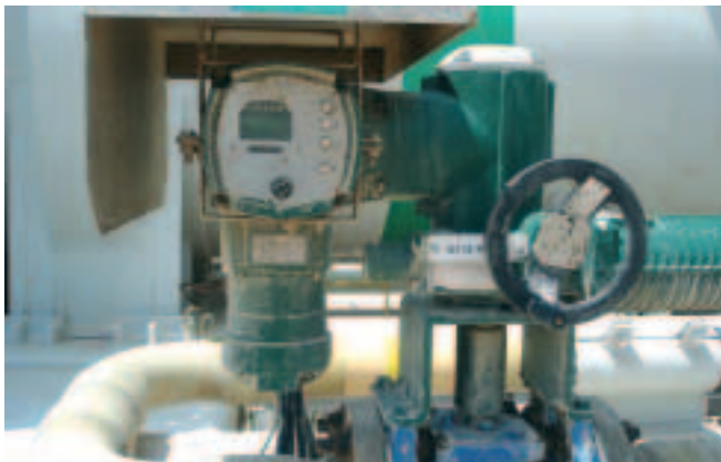
Applications under extreme conditions. SG part-turn actuator with AUMATIC in the Arabian desert in Qatar.
