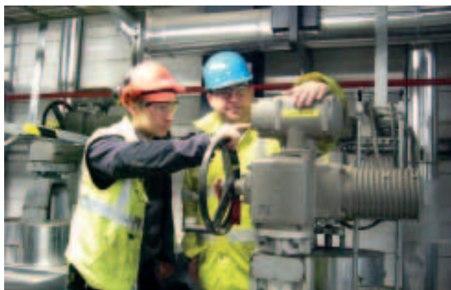
SA multi-turn actuator with AUMATIC on a gate valve in a peat-fired power plant in Ireland.
