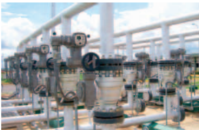
Explosion-proof AUMA actuators with AUMATIC at a tank farm in Venezuela
