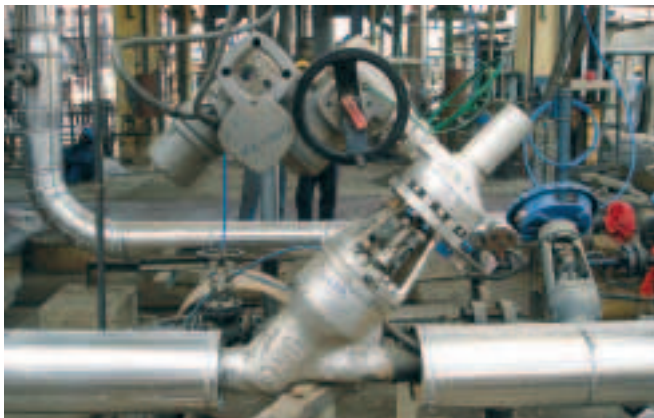
Fireproof version of an AUMA SA multi-turn actuator with AUMATIC – Devices with this coating remain fully operable for at least 30 min. if exposed to temperatures up to 1,100 °C in case of a fire.
