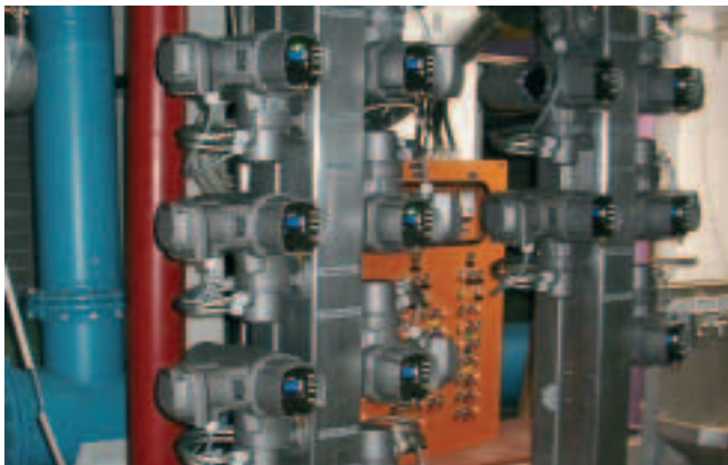
AUMATIC “collection” point within a water treatment plant. The controls are mounted separately from the respective actuators on wall brackets.
