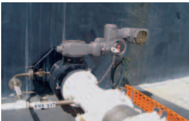
Explosion-proof SAE/C/GS multi-turn/part-turn actuator combinations with AUMA MATIC mounted on a butterfly valve within a tank farm in the Azores.
