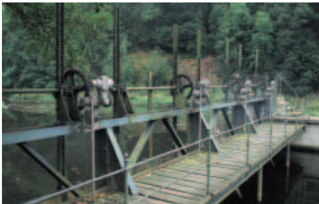
SA/GK multi-turn combinations with AUMA MATIC actuator controls integrated in a historical weir in East Germany.
