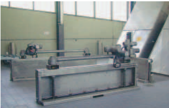
A number of double-stem gate valves in a sewage treatment plant. The combination between SA multi-turn actuators and GK multi-turn gear-boxes are each controlled by one AUMA MATIC.
